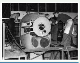
Top left, middle and right: All Halifax Merlin powerplants prior to the introduction of the Mk.II and Mk.V Series 1A had twin Gallay coolant radiators with single oval-shaped underslung Gallay oil coolers. The Gallay units were quite large and consequently also required rather bulky engine cowlings, the bottom edge of the radiator inlets featuring a noticeable forward rake.
