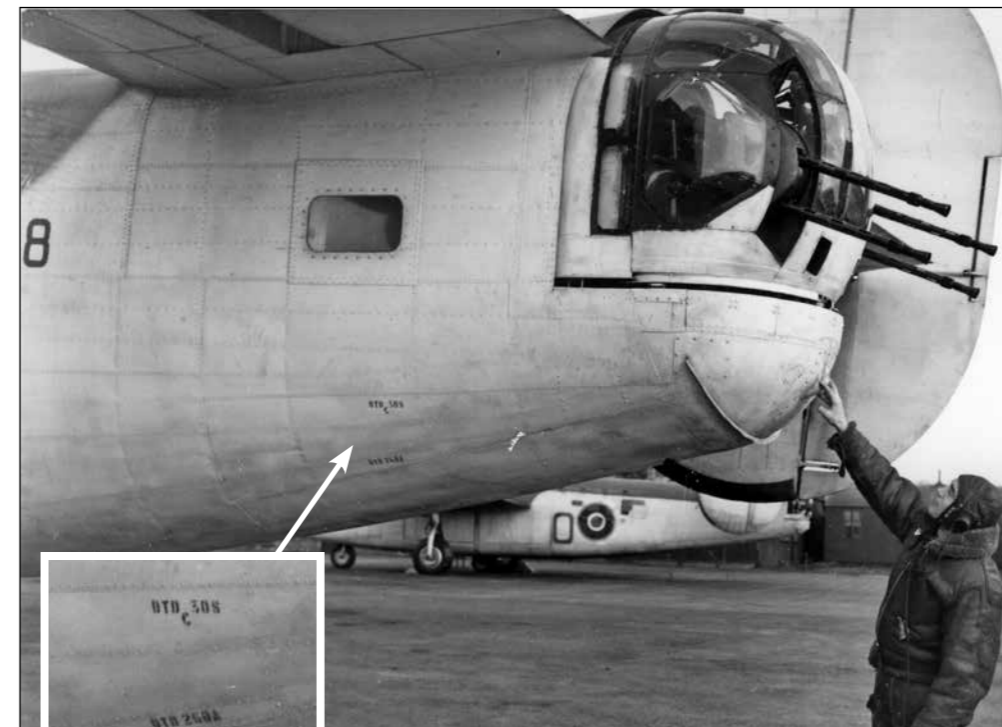
Above: The Boulton Paul Type E tail turret on a Liberator GR.Mk. III, 1943. This is the early version without the 'Clear Vision Sighting Panel' and defectors. The original black turret framing has been partially over-painted with white. The close up inset shows the DTD stencilling which describes the type of paint used, (DTD stands for Directorate of Technical Development).
